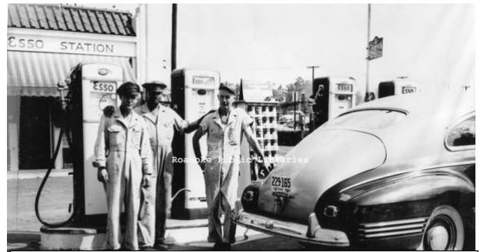
1940s Roanoke Esso Station, Roanoke Library
